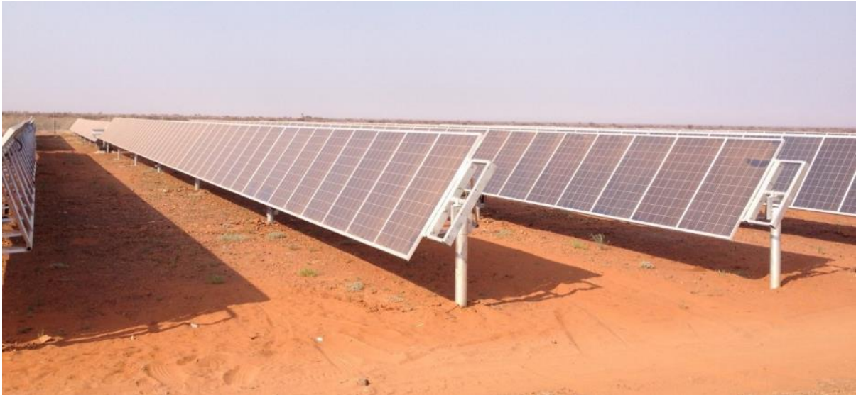
Figure 5-8: A single axis tracking system
